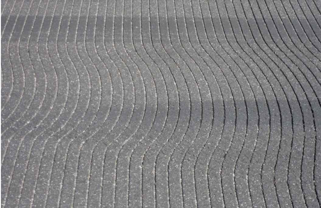
Figure 1. Typical cyclic shear creep failure.
