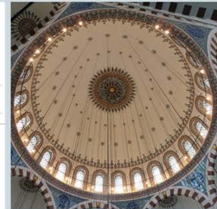
Rüstem Paşa Mosque Dome, Istanbul
