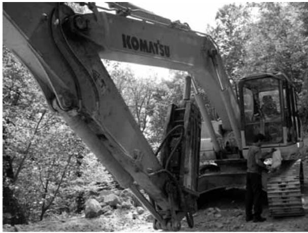
Fig. 2. Hydraulic hammer mounted to PC 220 Komatsu crawler excavator
