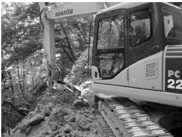
Fig. 4. Side casting of stones by hydraulic hammer
