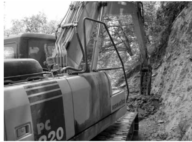
Fig. 3. Rock disintegration by hydraulic hammer
